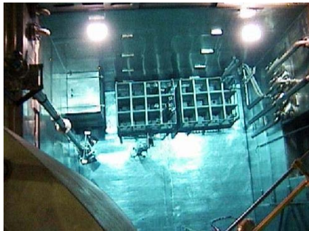
Figure 2. Storage racks in auxiliary pool of Peruvian reactor in Lima, Peru.
