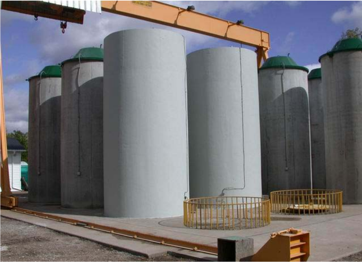
Figure IV: Canisters for storing waste from isotope production. Canisters in the background are used for storing spent reactor fuel.
