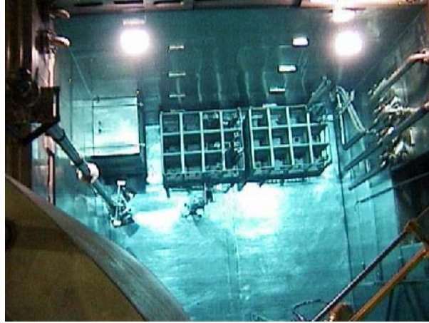
Figure 3: Storage Racks at RP-10
