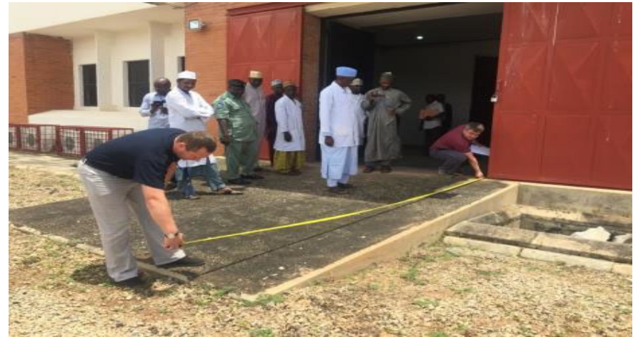
Outer and inner gates Ramp without a horizontal platform near the gate
