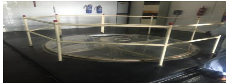
Reactor pool mounting on the floor
