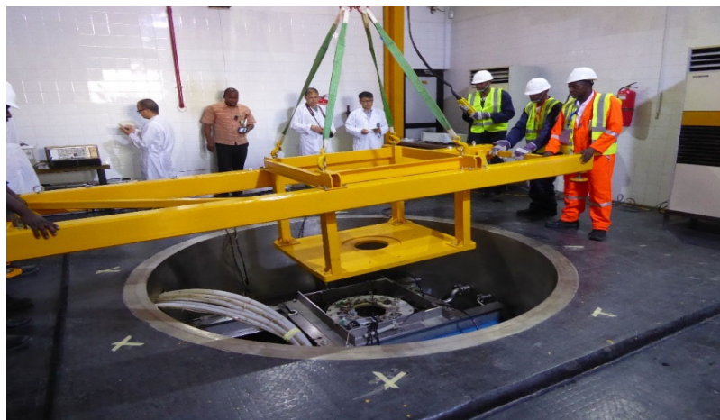
Equipment installation over the reactor pool
