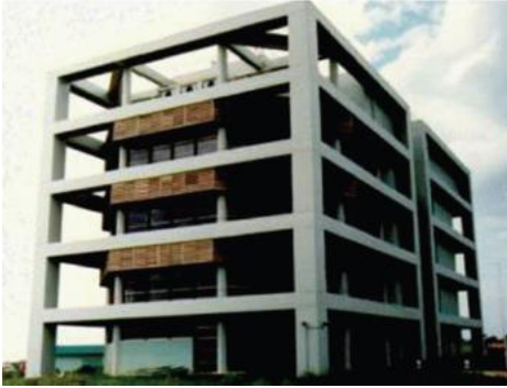
c) NUR reactor (Algeria). To be upgraded to 3.5 MWth [1], [2], [9].
