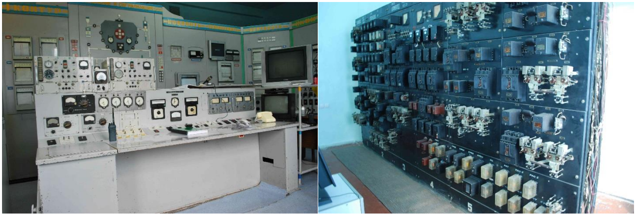
Pic. 3. Old control and protection system (CPS)
