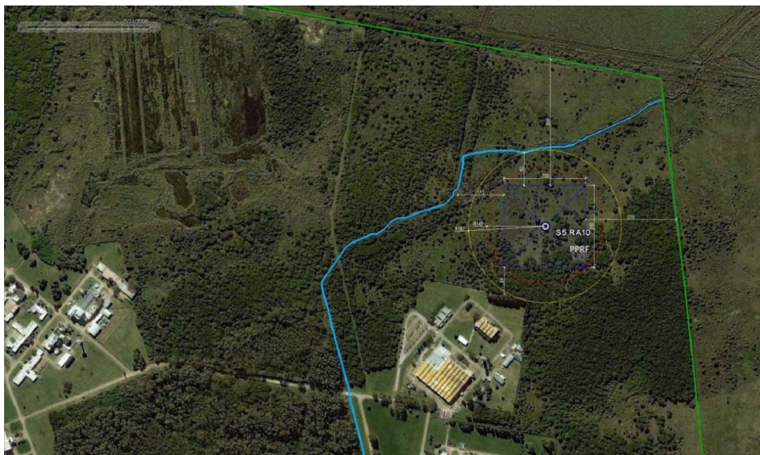
Picture n°1: PPRF and RA-10 location view
