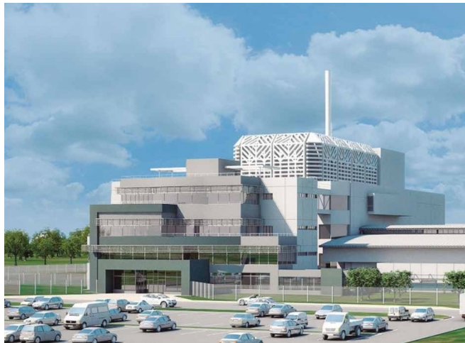
Picture n° 5: RA-10 front view
