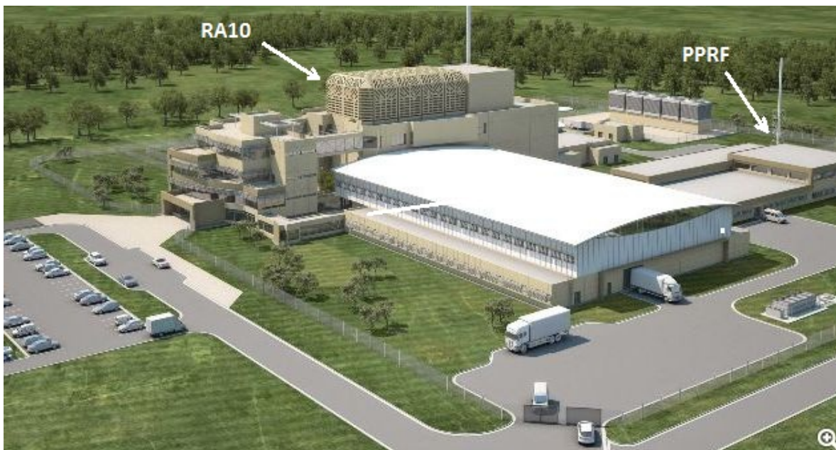
Picture n°3: PPRF and RA-10 lateral view
