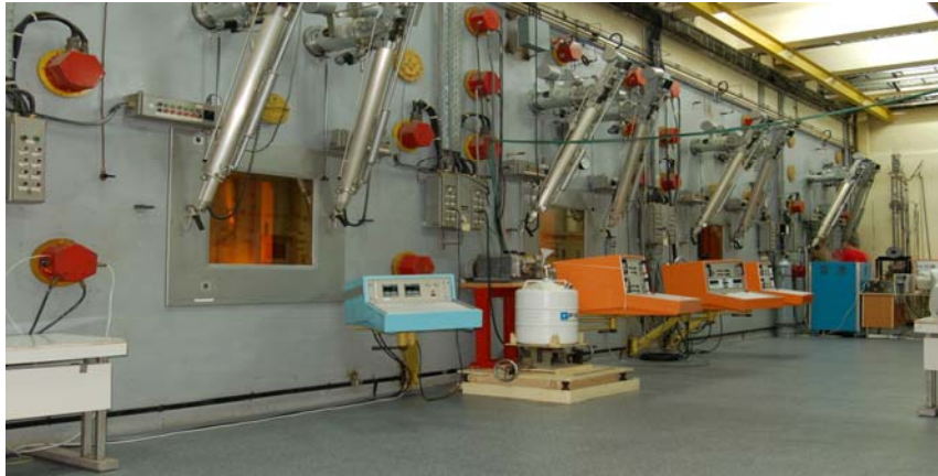
Fig. 6 Pitesti Reactor PIE Facility
