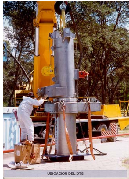
Fig. 7: DTS placed on top of ITS
