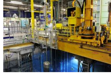
Fig.13: La Hague operator handling RRSF in HAO pool
