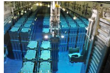
Fig.15: RRSF storage-basket transfer to wet storage
