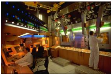
Fig.30: De-storage facility control room
