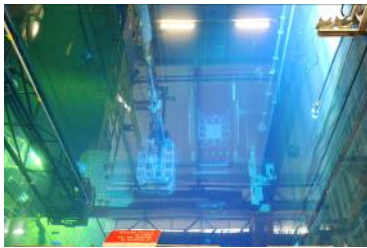
Fig.18: RRSF transfer from storage to shuttle basket
